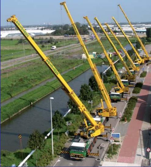
Dutch rental company Koninklijke Saan used seven Tadano Faun cranes to position a 425-metre long gas pipeline of 300mm diameter. Each crane took a load of 4.5 tonnes.
