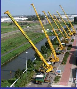
Dutch rental company Koninklijke Saan used seven Tadano Faun cranes to position a 425-metre long gas pipeline of 300mm diameter. Each crane took a load of 4.5 tonnes.
