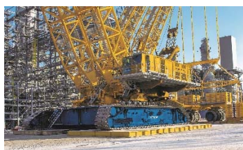
Demag Crawler Crane (CC 8800-1 TWIN)
