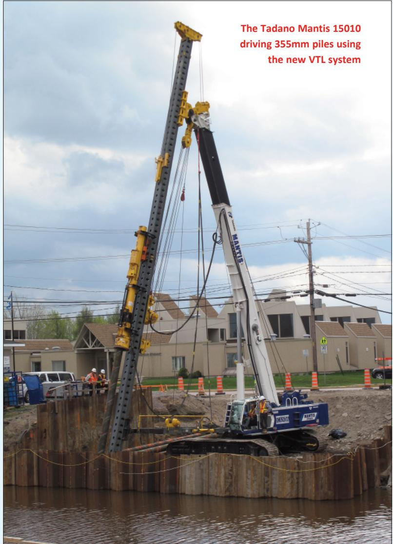
The Tadano Mantis 15010 driving 355mm piles using the new VTL system
