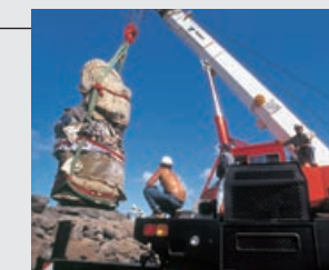
Moai Statue restoration project
