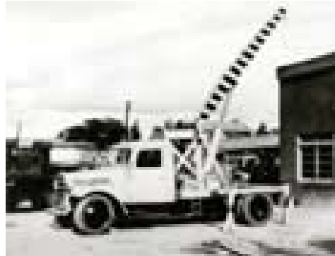
The OC-2 hydraulic truck crane
