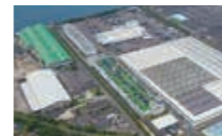
Solar panels installed at the Shido Plant
