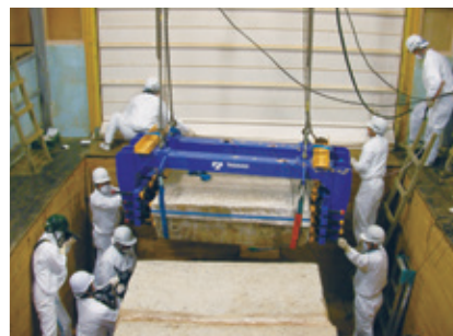
Disassembly of the Takamatsuzuka Tomb's stone chamber
