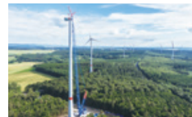
Assembling wind power generation equipment
