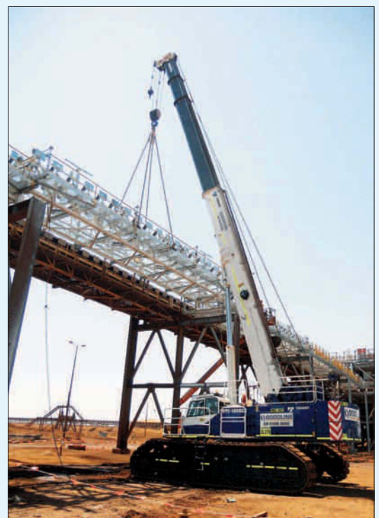
Goodline's GTC-1000EX builds Fortescue Metal's iron ore conveyor
