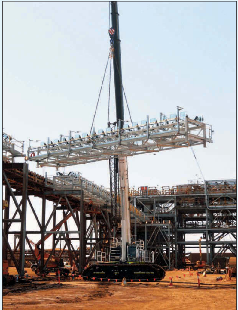
Goodline's GTC-1000EX builds Fortescue Metal's iron ore conveyor
