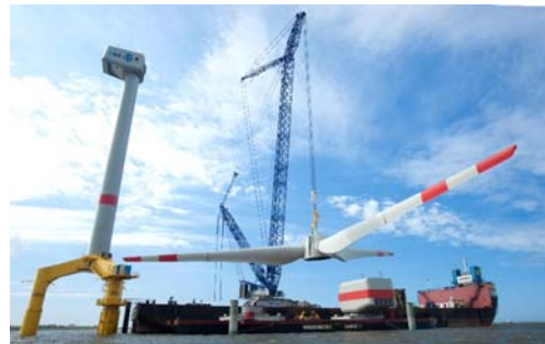
A crawler crane lifting the blades for assembly of an offshore wind turbine.
