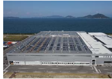
Solar power generating equipment on the roof of Kozai Plant
