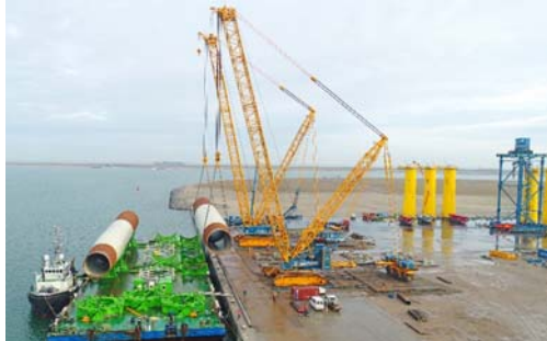
Crawler cranes loading offshore wind turbine components at a port.
