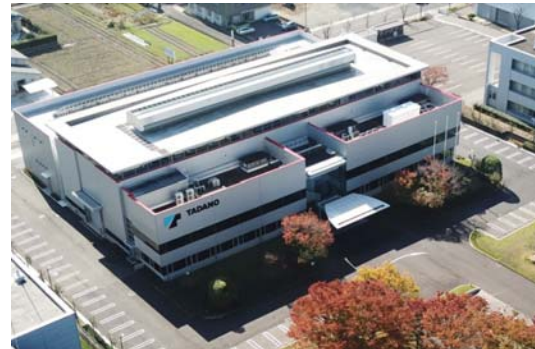
Expansion in 2020 of Tadano's Advanced Technology Research Center (In Takamatsu, Japan).
