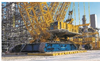
Demag Crawler Crane (CC 8800-1 TWIN)
