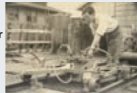
Railroad track maintenance machine
