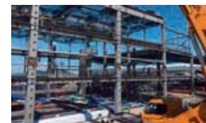
Power train testing facility under construction
