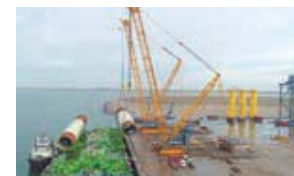
Crawler cranes loading offshore wind turbine components at a port
