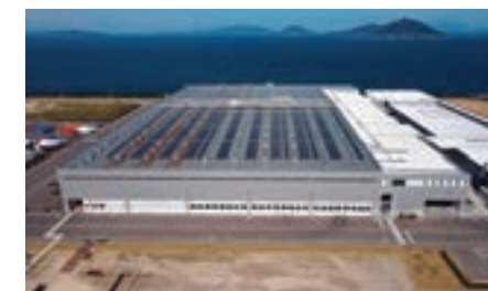
Solar panels installed at Kozai Plant
