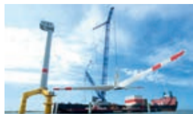
Assembling equipment in the harbor
