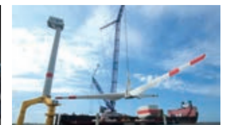
Assembling wind power generation equipment
