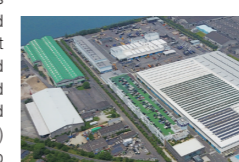
Solar panels installed at the Shido Plant
