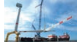
Assembling wind power generation equipment
